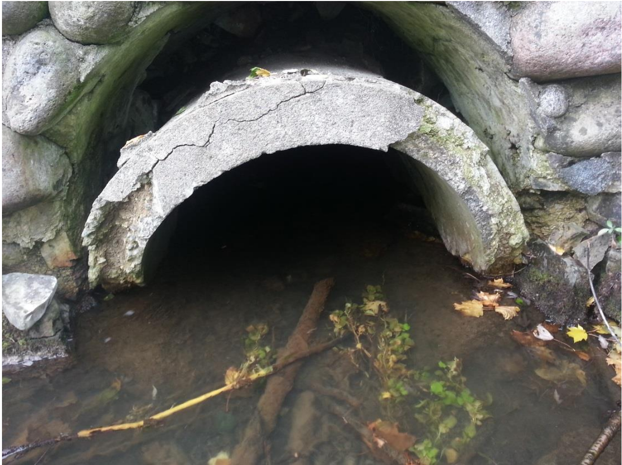
Figure 17: Degradation of Inlet of Culvert from site visit on October 30, 2014
